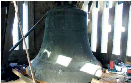
Glockenrenovation in Goldach
